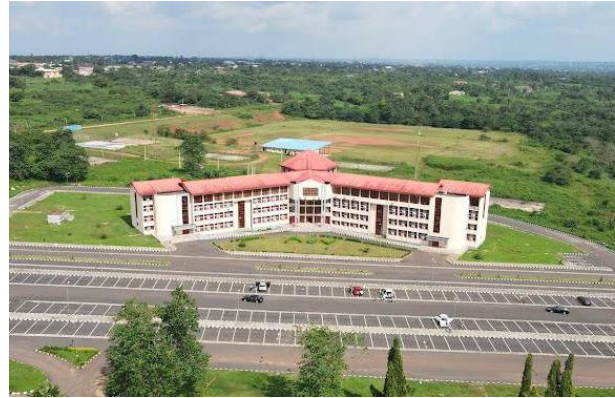
Figure 3. Aerial view of the location, Ambrose Alli University Ekpoma, Nigeria,(310103, 6°44.3'N, 6°04.9'E)
